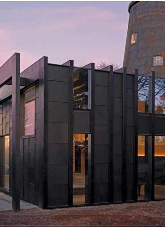
Jack Mill House
